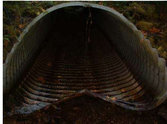
Reach 2 - Unit 208 Culvert - The end is crushed
