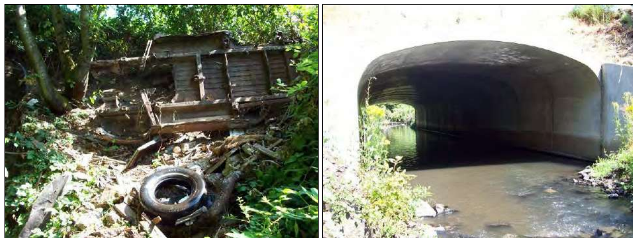
Figure 4-24. Debris such as old car bodies was used in the past for bank stabilization treatments (left). A concrete arch at SE 2 nd Avenue provides fish passage (right).
