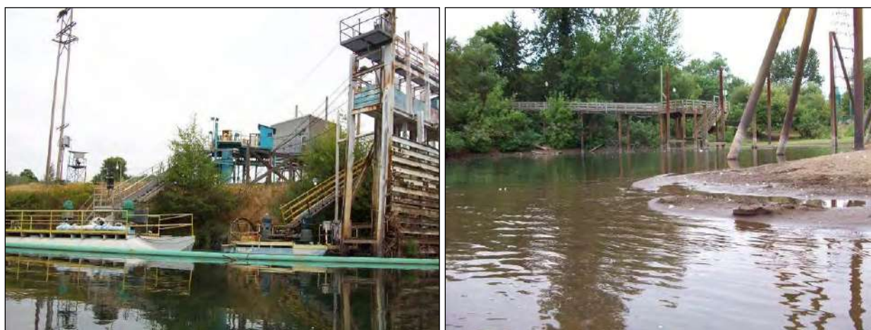
Figure 4-17. The pump station on the Willamette River supplies water to the ATI-Wah Chang facility (left). Pilings protect the City of Albany pier on the Willamette River downstream from the Calapooia River confluence.
