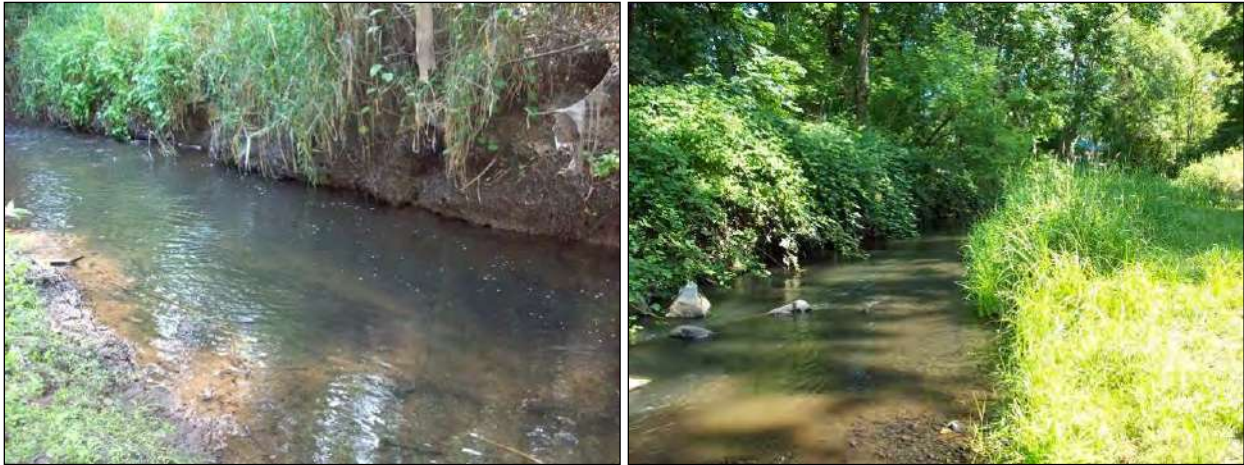
Figure 4-25. Example streambank erosion sites on lower Periwinkle Creek. The left photo is site E6, a river-left eroding site at STA 8+00. The right photo is from the E4 site located at STA 12+00. The river-left toe of the bank has been scoured.
