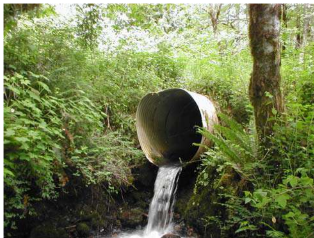
Fish passage barrier on a tributary to Brush Creek
