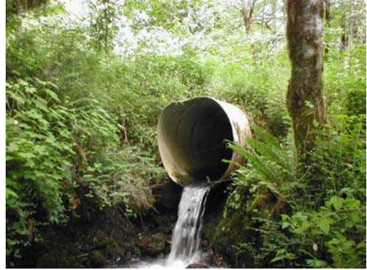
Photo 1. Outlet drop from a culvert located in the headwaters of Brush Creek. This outlet drop is greater than the jumping ability of fish.
