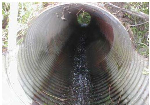
Photo 2. The inlet to a culvert located in the headwaters of Courtney Creek. This culvert has a steep gradient (12%) and shallow water that prevent fish passage.
